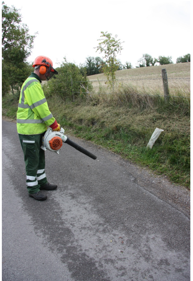
Highway inspections in the Pewsey area
